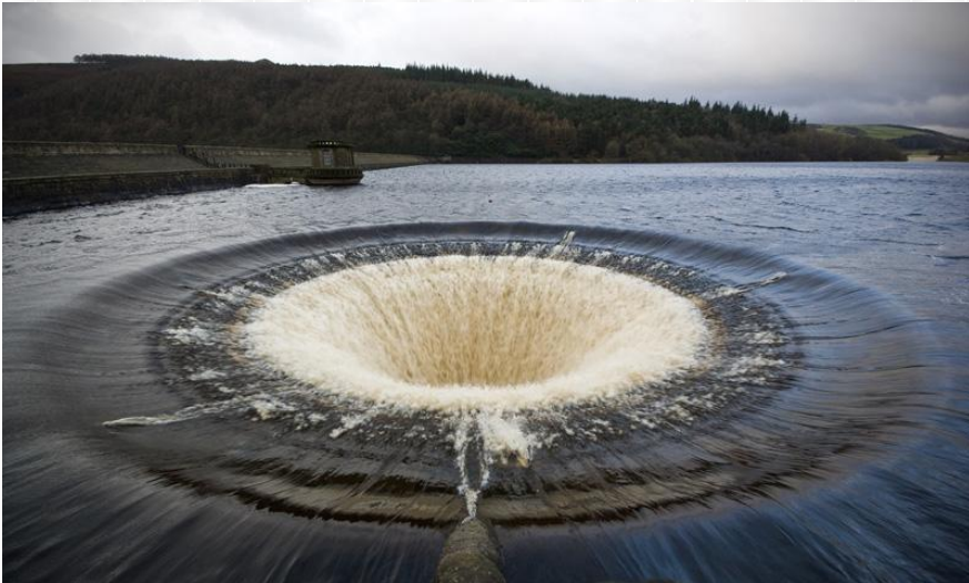
Bell-mouth spillway at impoundment Ladybower Reservoir.
